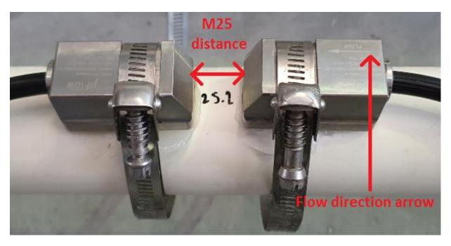
Note: The two transducers should be mounted at the pipe's centreline on horizontal pipes. Make sure that the transducer mounting direction is parallel with the flow. During the installation, there should be no air bubbles or particles between the transducer and the pipe wall. On horizontal pipes, the transducers should be mounted in the 3 o'clock and 9 o'clock positions of the pipe section to avoid any air bubbles inside the top portion of the pipe.
